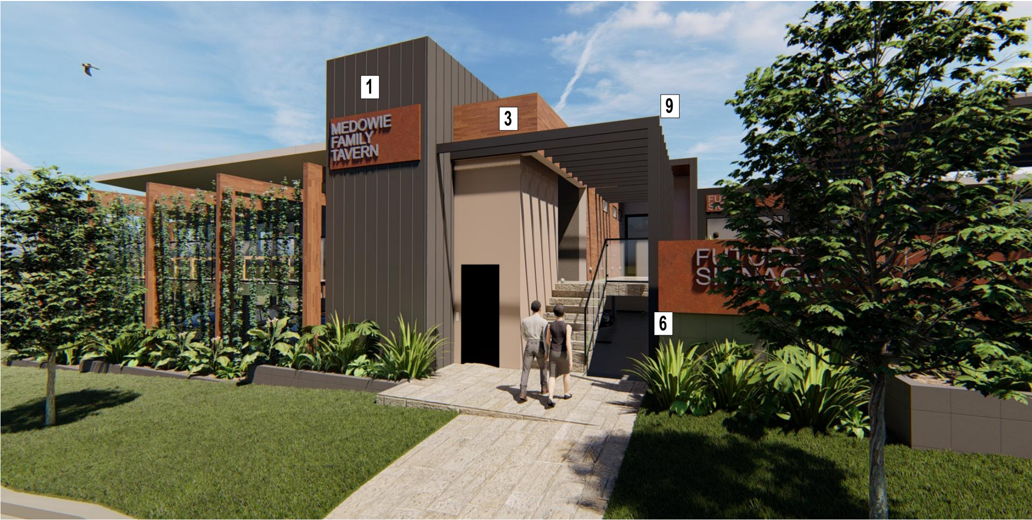
COLORBOND STANDING SEAM CLADDING
