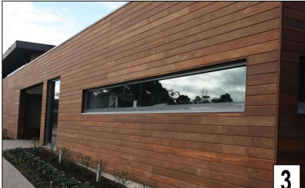
BLACKBUTT TIMBER CLADDING
