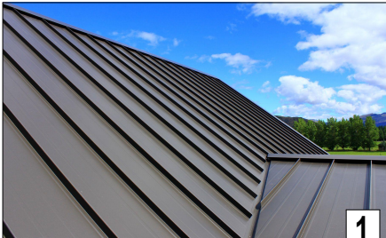
COLORBOND STANDING SEAM CLADDING
